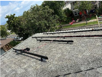
PV Racking and Arrays before and after panels are laid (all modules)
